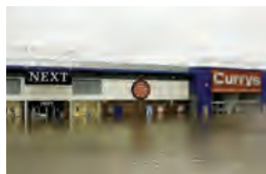
2007 floods submerged Chesterfield retail park causing damage to the stores and car park. Credit: Jon Bradbury.
