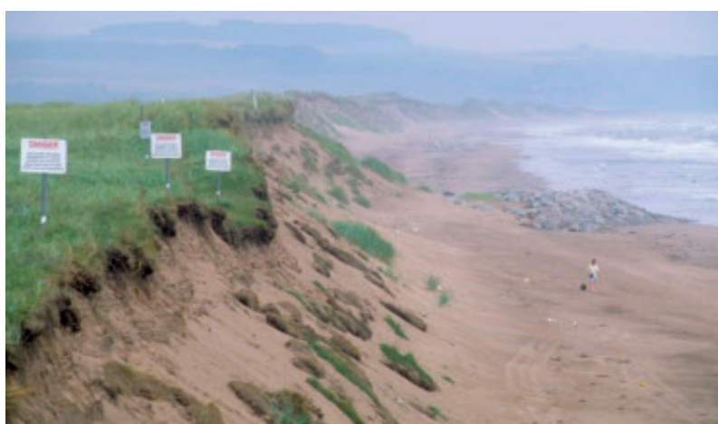
Coastal Erosion, Montrose
